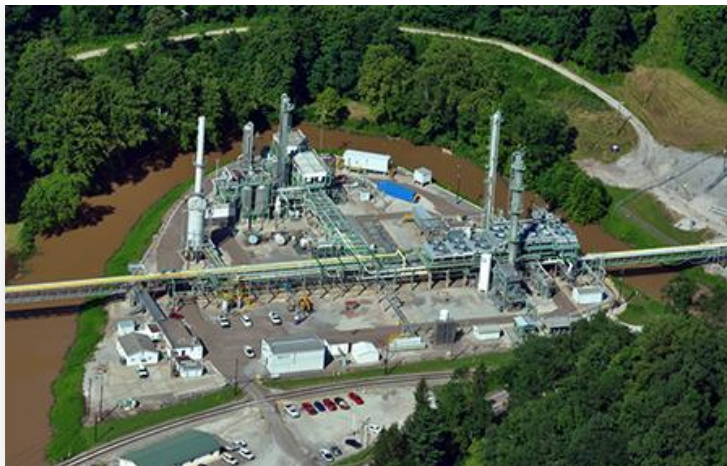
Gas processing plant. Photo courtesy of Bob Donnan.
